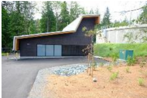
Reservoir #1 Electricity Generation Facility (Photo courtesy of City of Nanaimo)
