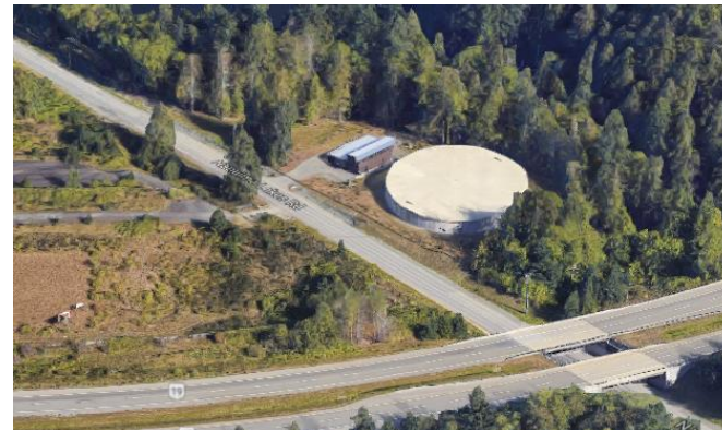
Overhead view of Reservoir #1 (Screenshot courtesy of Google Maps)
